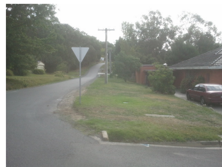
PHOTO 2 VIEW OF EXISTING HOUSE & GARAGE ALONG CRESCENT ROAD
